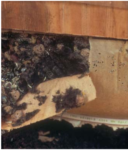
Fig. 10. Insulation in a wall space filled with dry dog food pellets and sunflower seeds. Mice gathered and stored the food, which caused a serious cupboard beetle infestation in the house. Note the beetle holes in the insulation paper in the upper right corner.
