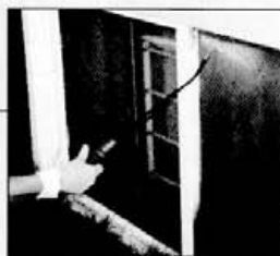
An example of a proper spray application beneath the lower edge of siding.
