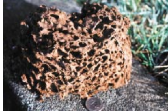
Fig. 8b. Moisture ant galleries made from damaged pressboard.
