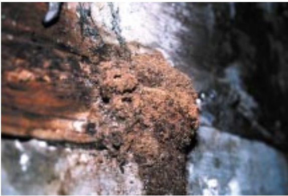
Fig. 8c. Moisture ant colony on a mudsill in crawl space.
