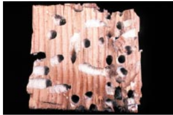
Fig. 9. Teredo or shipworm damage.
