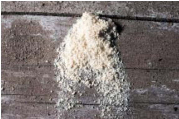
Fig. 4c. Anobiid frass expelled from hole.
