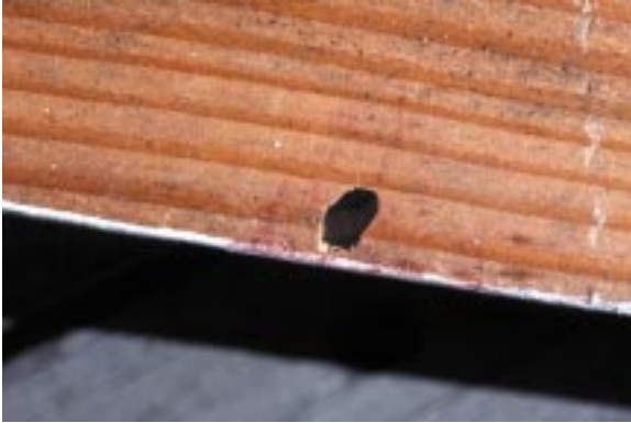
Fig. 5a. Buprestid beetle exit hole.
