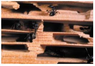
Fig. 3. Typical carpenter ant damage.
