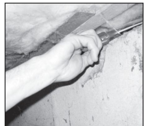
Inspecting for termite damage.
